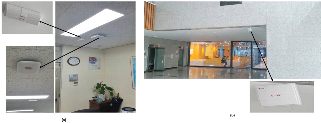
Fig. 13. Small cells (SC) deployed within the center as mmWave solution, where (a) LGU+ and Samsung electronics SC and (b) LGU+ SC deployed at the center.
